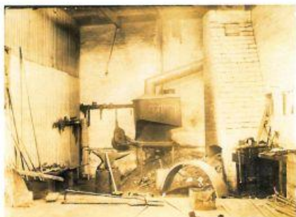
Jackson and Jones arrived in Sydney in 1912 and operated at 364 Parramatta Road Petersham, the premises of the Surrey Cycle & Motor Co., during the period 1913 to 1917. Top left: The blackboard was used for full-size drawings, from which the body builders could take measurements. Left: The smith's furnace for making the ironwork for the bodies. Top: The 'Jackson & Jones Motor Body Builders' sign above the door with it is thought Harold Jackson. Below: A 'Jackson & Jones' body plate from this era.
